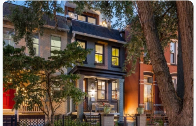
NetZero Rowhouse Teass \ Warren Architects
